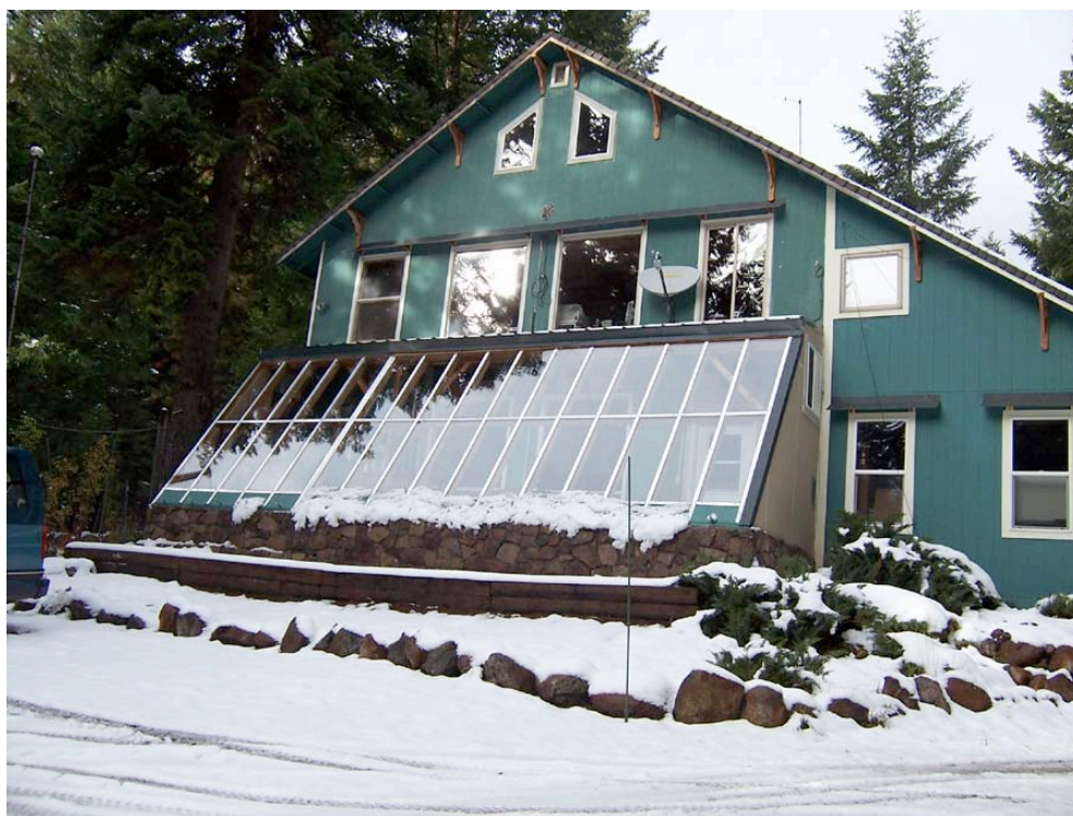
South-facing wall of the OBRL Laboratory/Seminar Building with new Passive Solar Heating System/Solarium.
